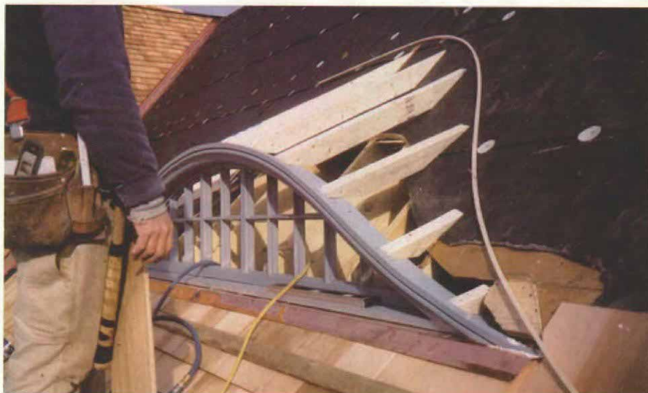
Simplified framing, too. The eyebrow dormer was framed with 2x4 rafters, and the curved jamb was used as a header. Because the window looked out from an unfinished attic, the roof rafters behind it could be left intact. A pine batten is being used here to lay out a fair curve on the main roof.
