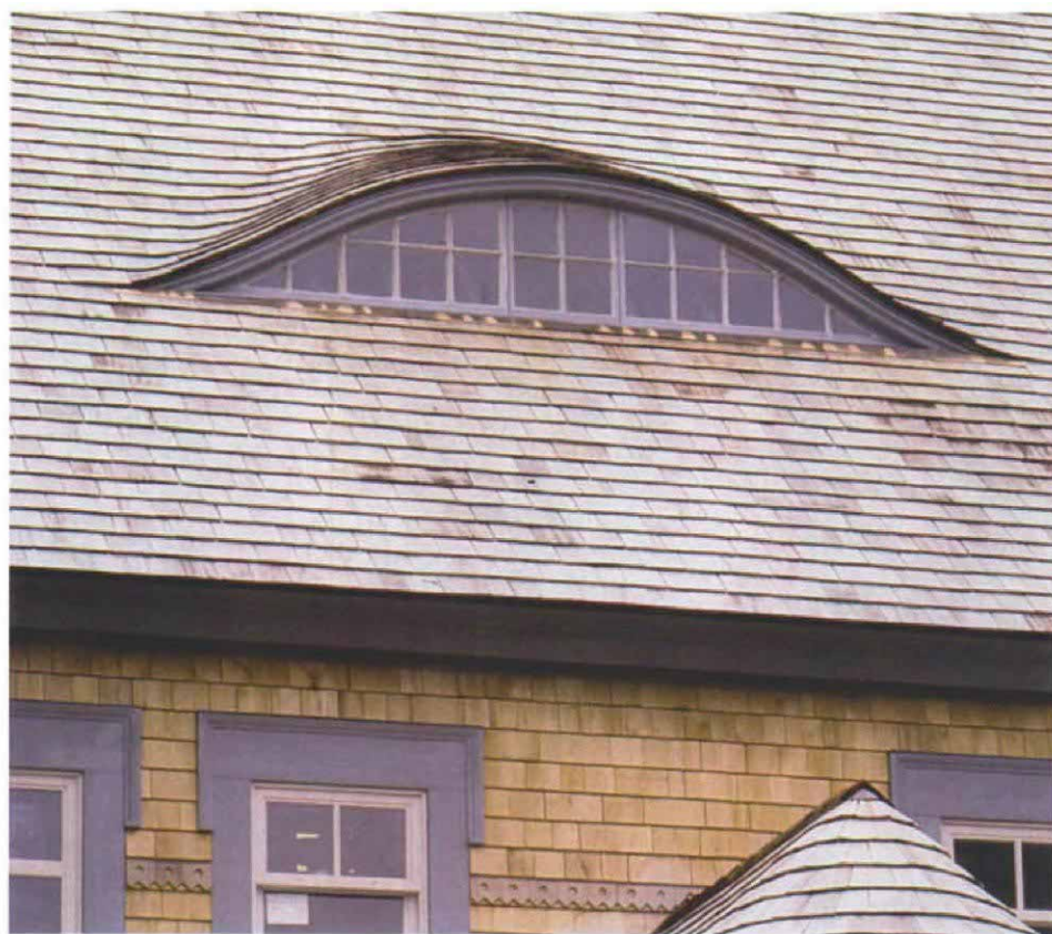
An unexpected curve. Lap joinery, used by the author to build this eyebrow window, offers an alternative to cope-and-stick joinery. Photo by Charles Wardell.
